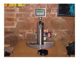
The taps are centrally supplied from cooled beer box, where is the beer kept in 3000 litters beer tanks. The non pasteurized beer is kept in plastic sack, which is placed in the tank and is pushed out, using the air, which occurs in the space between the rustfree wall of the tank and the plastic sack. The beer does not come into straight contact with driving gas, which means, it is of higher quality. The beer sub-cooled all the way to every single table.
